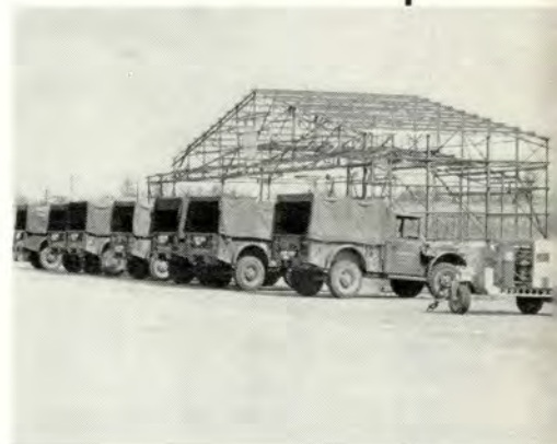
During test there were no ground or air accidents—no incidents occurred.
